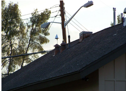
Image 5: After the instal the pigeons stopped landing on the roof.
